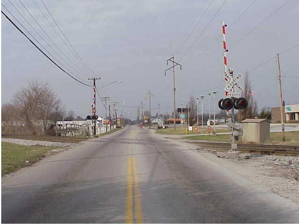
479854T-09162009-02.jpg - - W Side of Xing; Hwy Approach looking E
