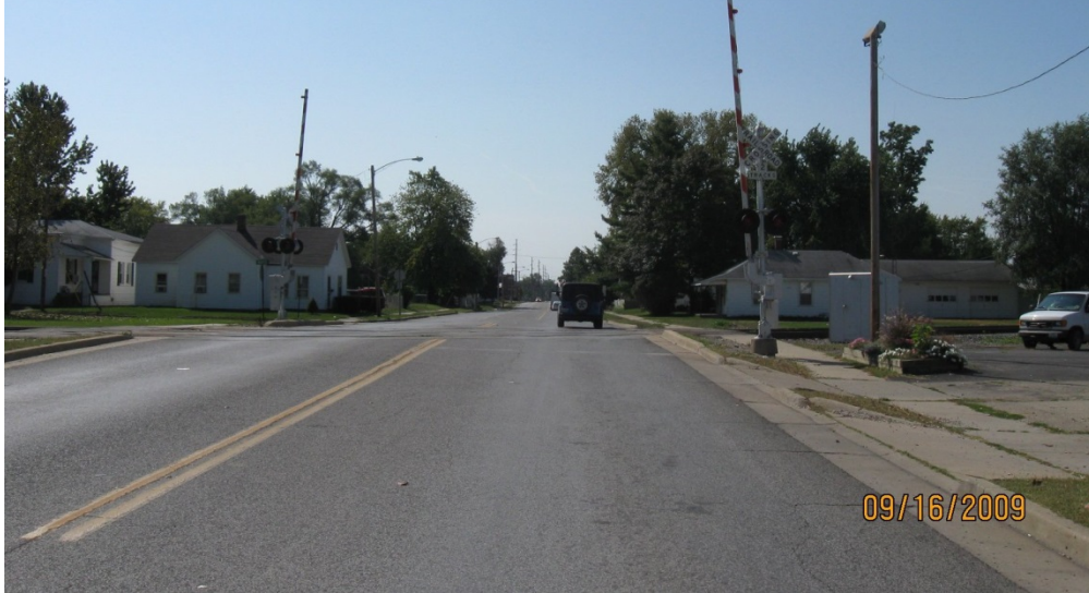
479856G-09162009-07.jpg - - S Side of Xing;Hwy Approach looking N
