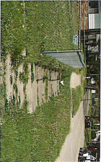
Some blocks appear to have “disappearing sidewalks” where weeds and lawn have begun to grow over failing concrete
